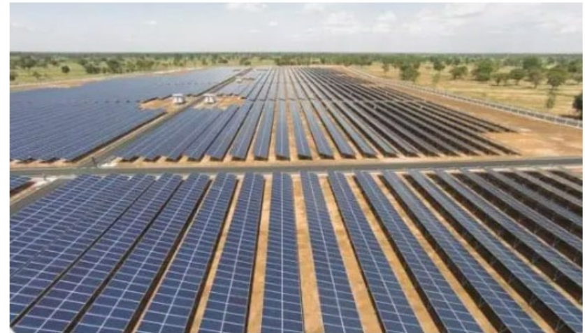
Bungala solar farm.
